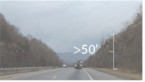
Large Cut, Sloped Embankment
