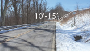
Sidehill, Sloped Embankment
