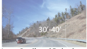
Large Cut, Sloped Embankment
